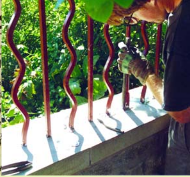
Installation and restoration of railings at the front of Park Hill.
